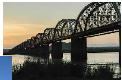
Dona Ana Railway Bridge Zambezi River – 3,7 km (1934)
