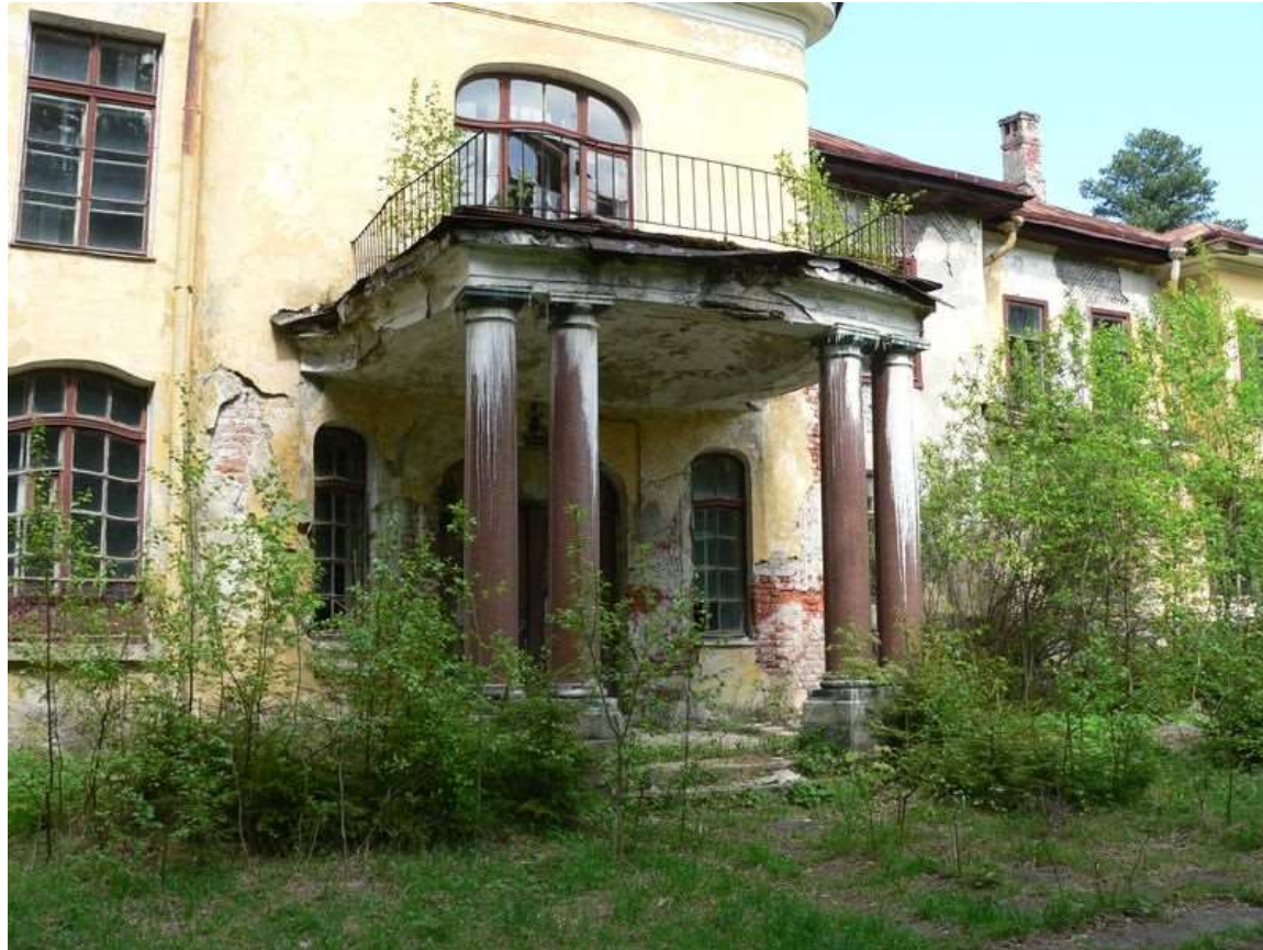
Agathon's former country house, Levashovo, now in a ruinous state
